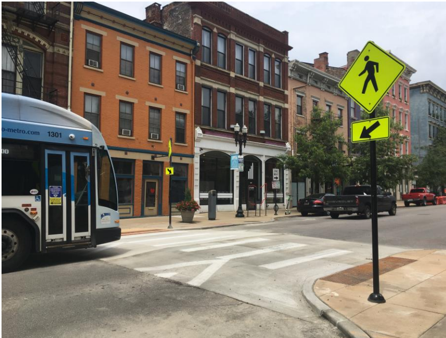
Raised crosswalk at Main & Orchard Streets
