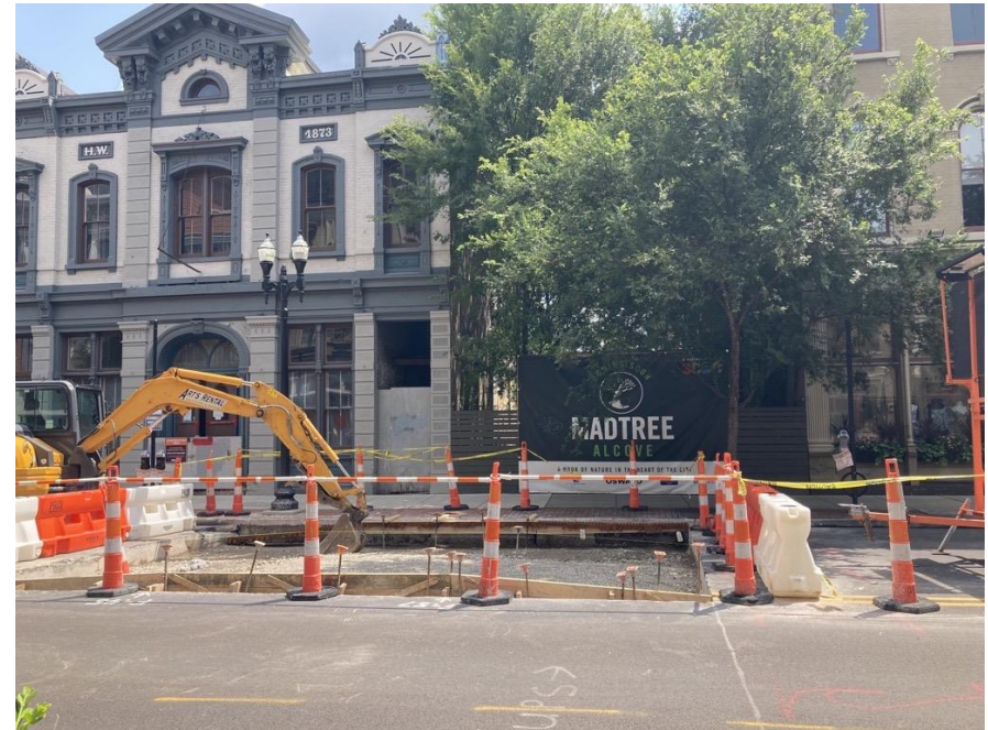
Vine Street – under construction
